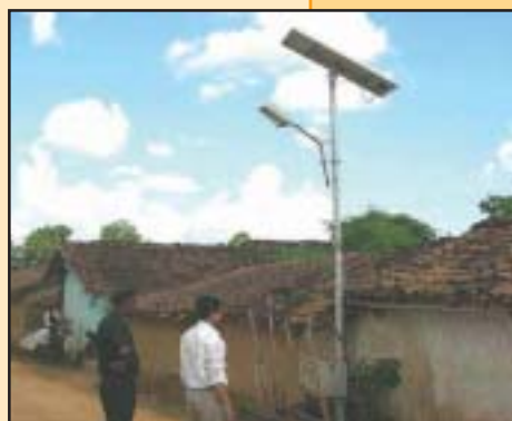
Solar Street Light
