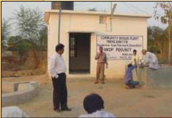
Community Bio-Gas Plant in Mahulbhatta village of Komna block
